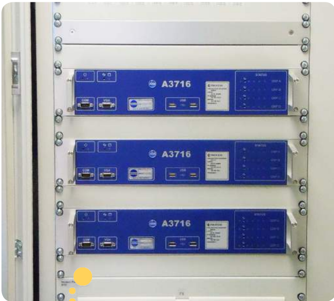
Example using 3 pieces of A3716 2U monitoring system on site
